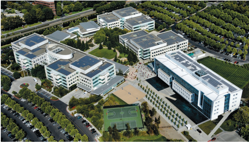
eBay's solar power system.
